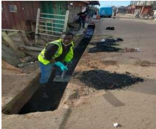
Drains being desilted during the clean-up exercise at Beraku
